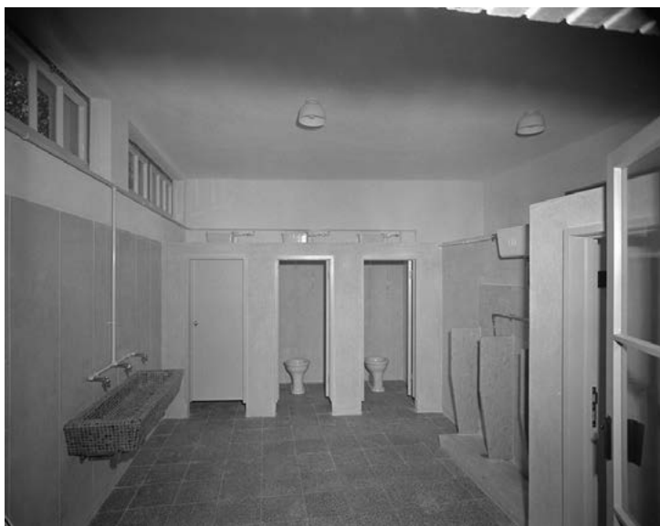
Figure 54 Toilets at Escola Primária N.º 63, in Restelo, photograph by Armando Maia Serôdio, 2 October 1958. AML, PT/AMLSB/CMLSBAH/PCSP/004/SER/001834.
