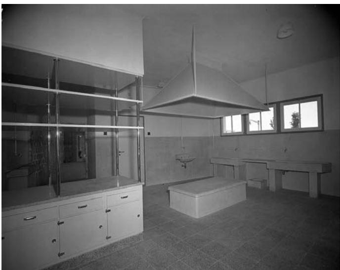
Figure 49 Kitchen of the canteen at Escola Primária N.º 63, located in Praça de Goa, in Belém, photograph by Armando Maia Seródio, 2 October 1958. AML, PT/AMLSB/CMLSBAH/PCSP/004/SER/001831.
