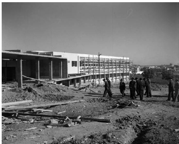
Figure 36 Visit by Lisbon Municipal Council to the construction site of the Grupo Escolar da Célula VII in Alvalade, now Escola Básica do 1.º Ciclo do Bairro de São Miguel, located in Rua Jorge Ferreira de Vasconcelos, photograph by Armando Maia Serôdio, 28 October 1954. AML, PT/AMLSB/CMLSBAH/PCSP/004/SER/000794.
