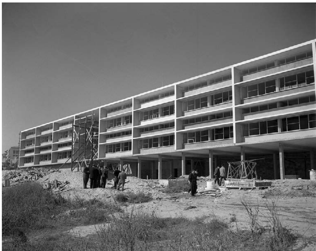
Figure 38 Visit by Lisbon Municipal Council to the construction site of the Grupo Escolar do Bairro de Santos, now Escola Básica Mestre Arnaldo Louro de Almeida, located in Rua Diogo de Macedo, photograph by Armando Maia Serôdio, 28 October 1954. AML, PT/AMLSB/CMLSBAH/PCSP/004/SER/000797.
